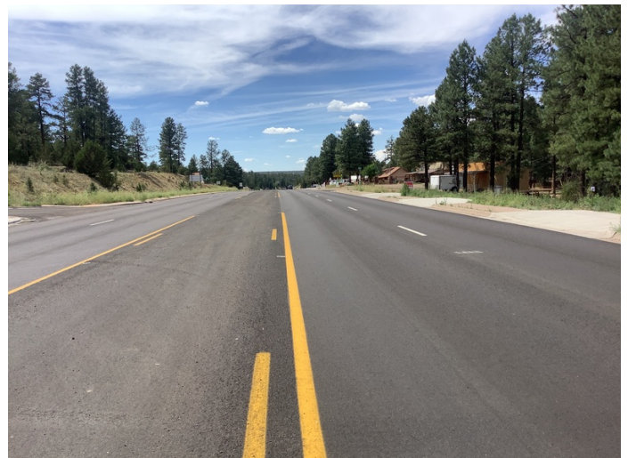
Completed project on SR-260 in Arizona
