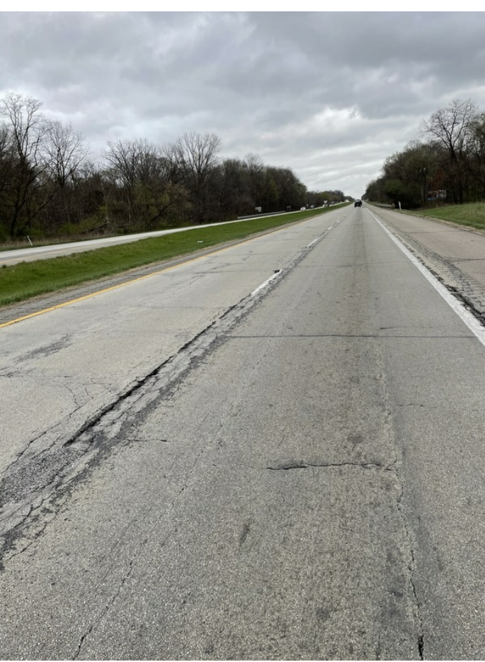
Existing Pavement Surface during Investigative Sampling
