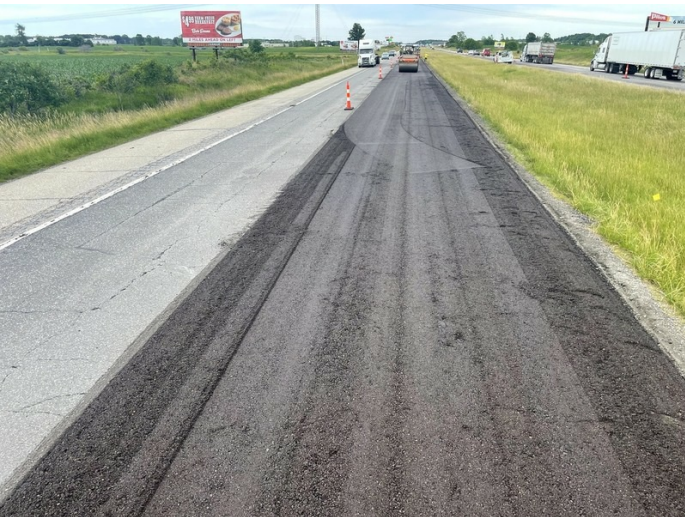
CIR was performed in phases by travel lane
