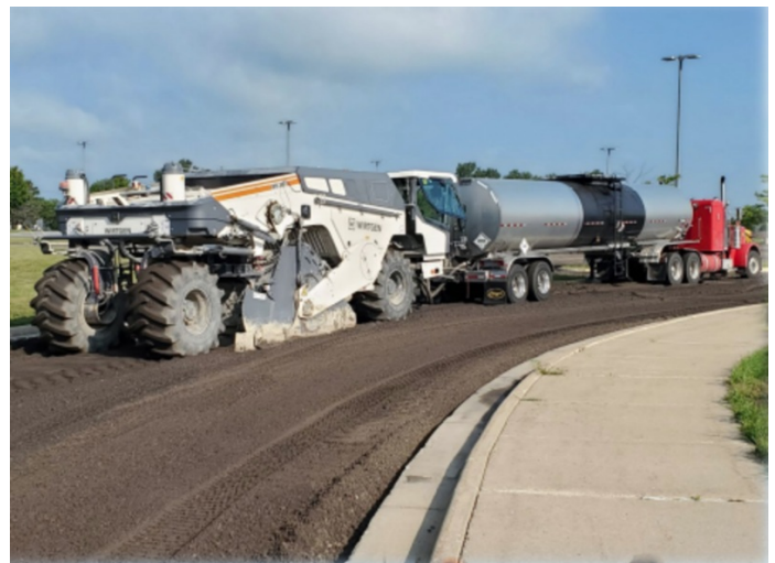
Performing FDR with emulsified asphalt
