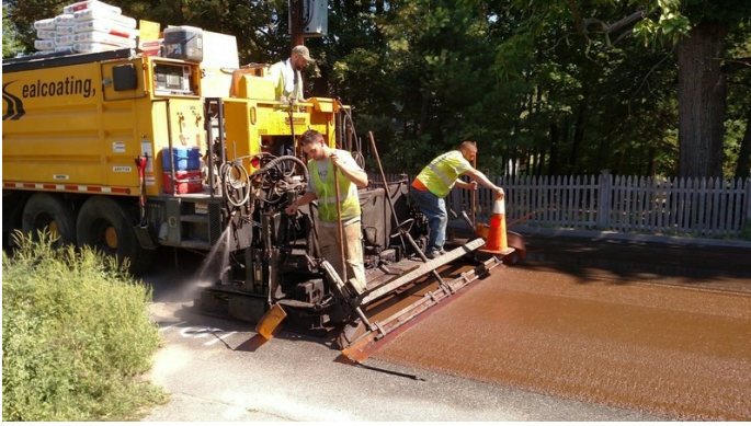
Application of Microsurfacing
