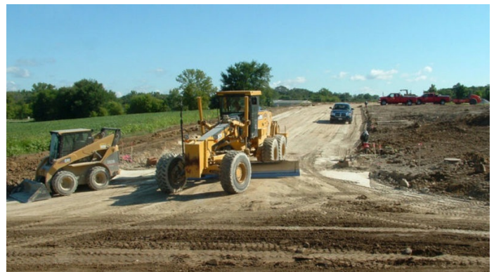
Final grading to elevation
