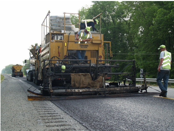
Micro Surfacing is applied over an entire 12-foot lane in a single pass.
