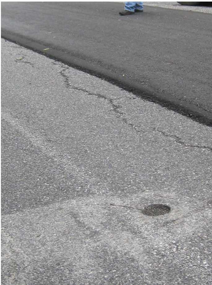
Existing asphalt and new asphalt base after recycle
