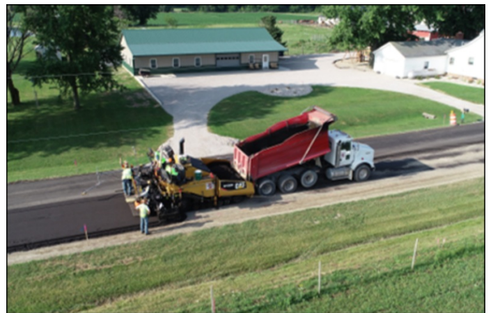
Paving of the 6.0-inch CCPR lift
