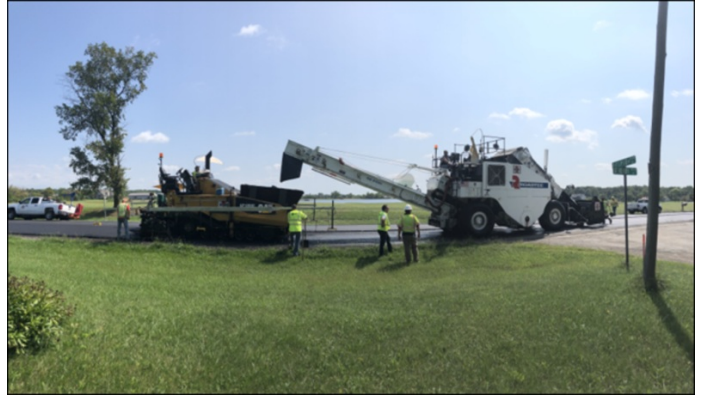
Paving of the 2.0-inch 12.5mm HMA surface
