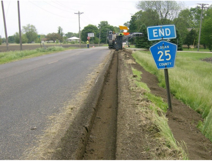
Trenching Material for Widening with FDR
