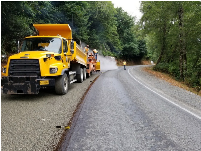
Chip seal in process
