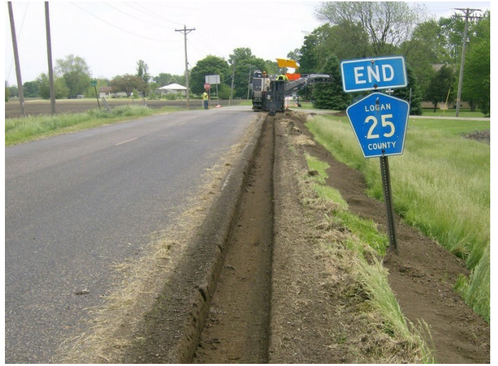
Trenching Material for Widening with FDR
