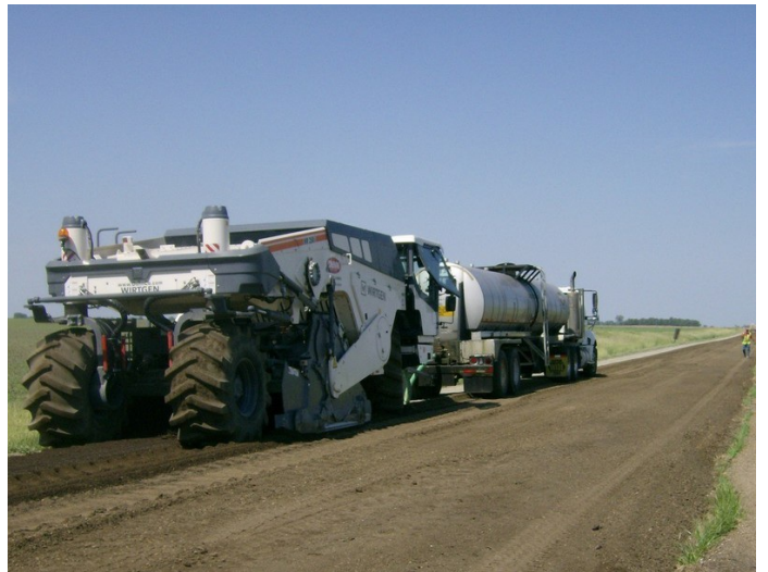
FDR Stabilization with Engineered Asphalt Emulsion
