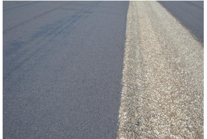
Installing the Micro Surfacing
