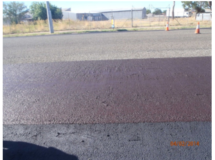
Installing the Micro Surfacing
