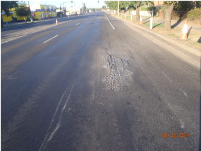
Pre-existing Condition - January 2014
