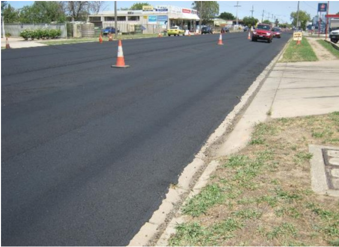
Installing the Micro Surfacing
