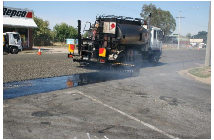
Installing the seal February 2014
