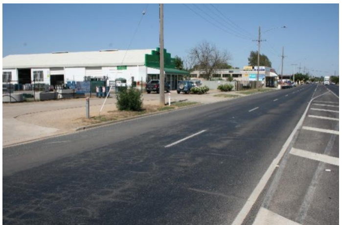
Pre-existing Condition - January 2014
